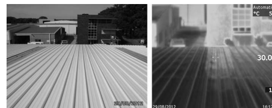
Figure (16). Visual and thermal images of the roof after the cool material application (2nd phase).
