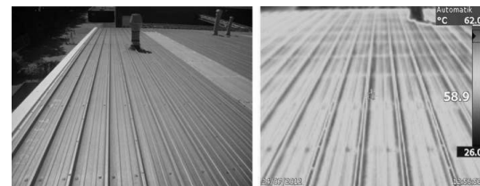
Figure (14). The roof before and after cool material application.
